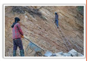
Therefore, a group of our regular construction workers are provided with the task to build a stone and concrete wall. The wall will prevent any debris from falling and reaching the school playground and avoid risking anyone standing in the vicinity. The work has already begun and is expected to be complete within a few weeks.
