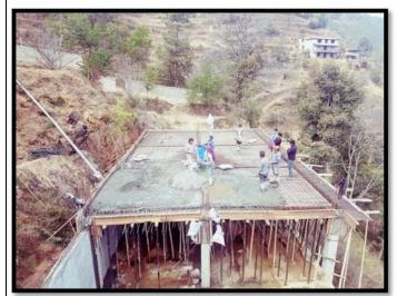
Garage Construction is on its peak. The sharing wall has been done. Pillar has construction been finished. Upper fundament for concrete slab (RCC) has been currently going on. There are total four workers and are staying at school and working. Their accommodation and lifestyle are very simple and is managed by Arjun, our contractor. It everything goes all right then this big construction will be finished within three months.
