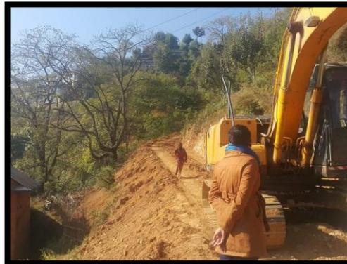
There are many challenges regarding the landslide area and garage construction. The stones, which were swept away by landslide, are still on the steep area. It is really risky with life of the workers working there. Hence, Arjun has called the digging machine to pull the stones up on the ground and can be manageable by workers.
